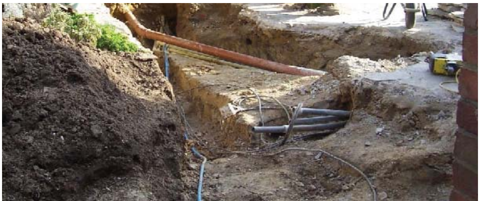
Excavations during the clean up of a spill
